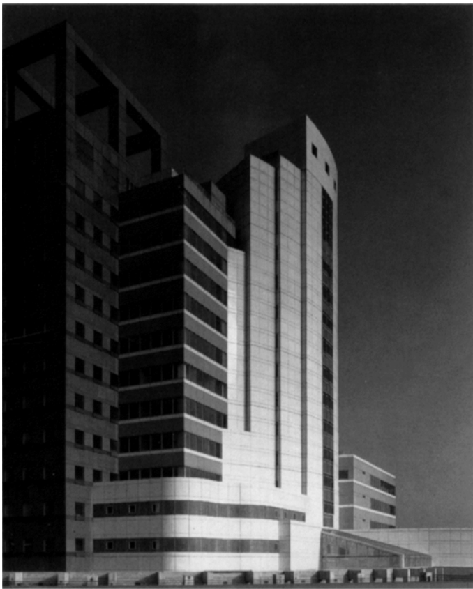
4. View of the southeast side from the roof terrace of the parking garage. (Photograph: Jeff Goldberg/Esto © 1989)
